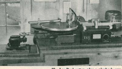
The Les Paul cutter, plus a playback arm. The two flat slabs under motor and cutter are iron plate.
